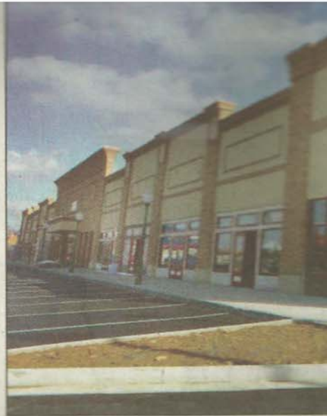
Most of the exterior work has been completed on the new retail building at Suncrest Towne Centre.
